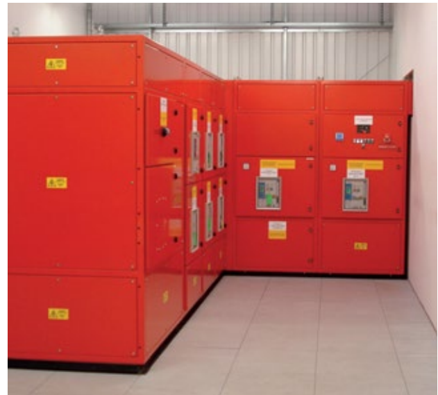
Figure 14 – Switchboards installed into the 12MW data centre which incorporated 3C overheating protection
