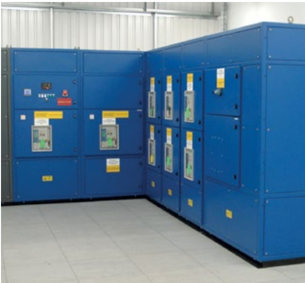
Figure 14 – Switchboards installed into the 12MW data centre which incorporated 3C overheating protection
