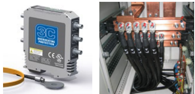
Figure 10 - External 3C module for busbar zone monitoring
